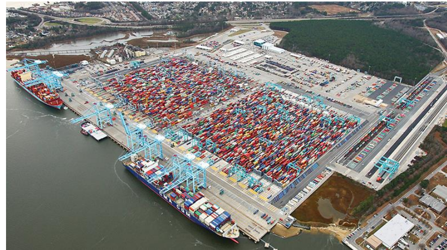
Aerial view of VPA's expanded Virginia International Gateway Terminal
