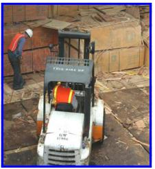
Make sure that steel plates are secure when a lift is operating in the hatch. If not the plates may shift
