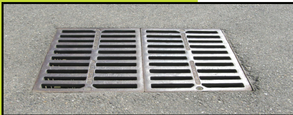
Dual Storm Drains
