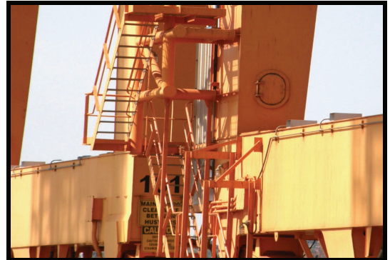
The Access to Crane Legs are considered confined spaces.
