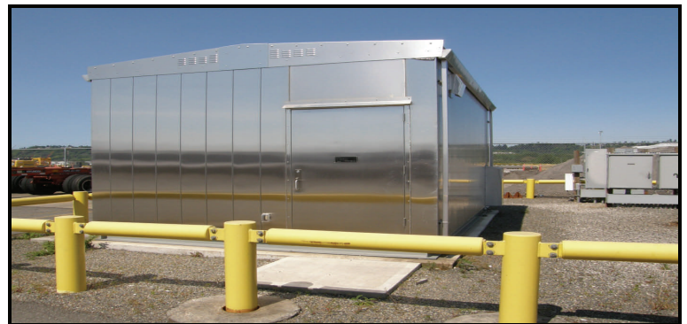
Another confined space could possibly be Electrical Rooms at Substations
