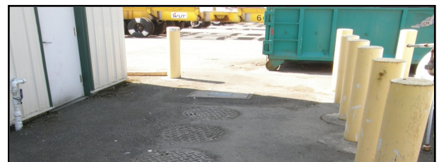
Vaults for Valves and Pumps at Wash Down Stations for Refer Units
