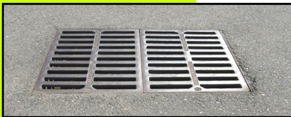
Dual Storm Drains
