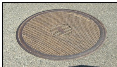
Electrical or Communication Vaults
