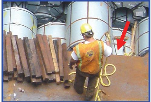
*Housekeeping plays an important roll in ensuring a safe workplace. Dunnage, can get thrown up by the lift, if not picked up*
